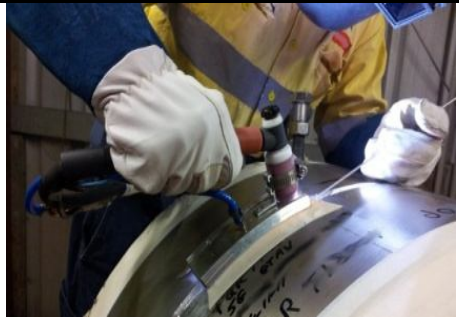
TITANIUM TIG WELDING
